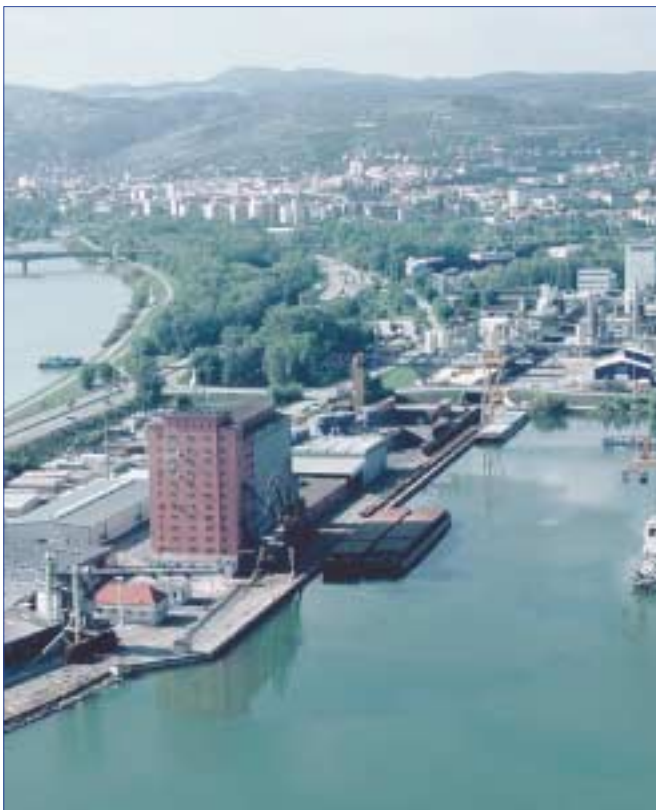
Krems Harbour at the Danube: Sustainable transport systems next to an UNESCO heritage site (co-financed by EC)
